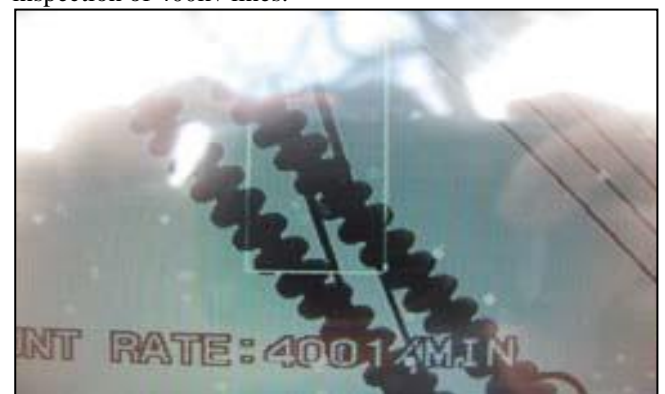
Fig. 4. Corona Inspection of 400kv lines
