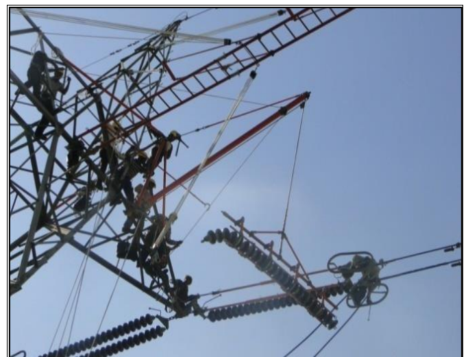
Fig. 8. Replacement of insulator string
