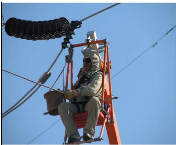
Fig. 9. Replacement of Jumper
