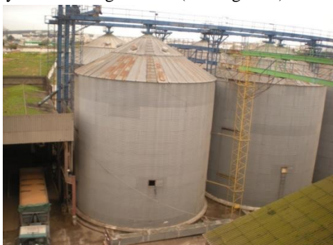
Figure 1: Metal storage infrastructure of grain silo
